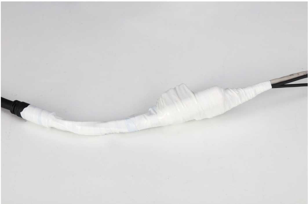
Figure 1-3 Covering exposed parts
